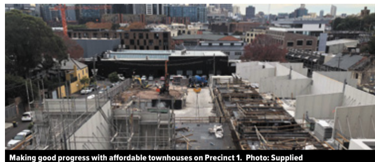
Making good progress with affordable townhouses on Precinct 1. Photo: Supplied
