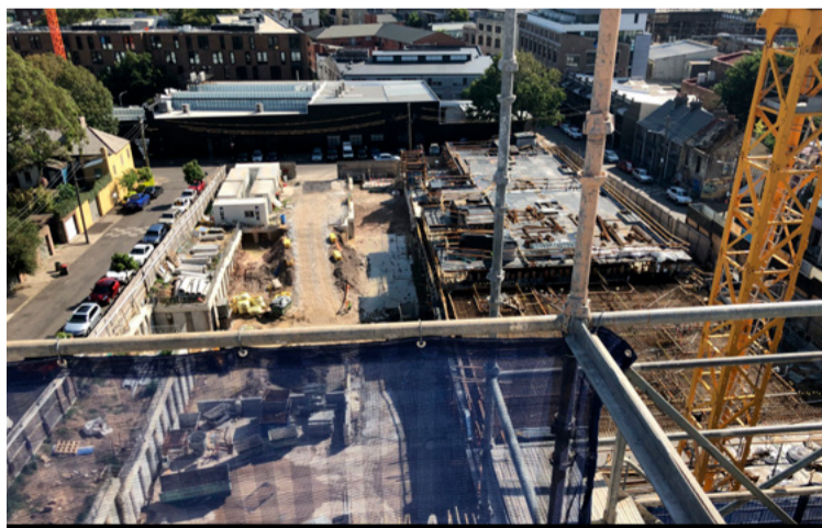
In March, further work on the Level 2 formwork for townhouses that face Eveleigh Street continued. The underground carpark can still be seen on the Louis Street side where the rest of the 62 townhouses will be built. Photo: Supplied – Taken from the vantage point of the upper level of the building housing 26 apartments above the Tony Eloura Gym which has reached its full height.
