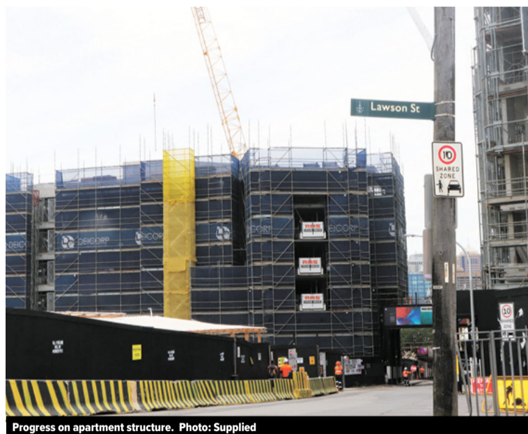
Progress on apartment structure. Photo: Supplied
