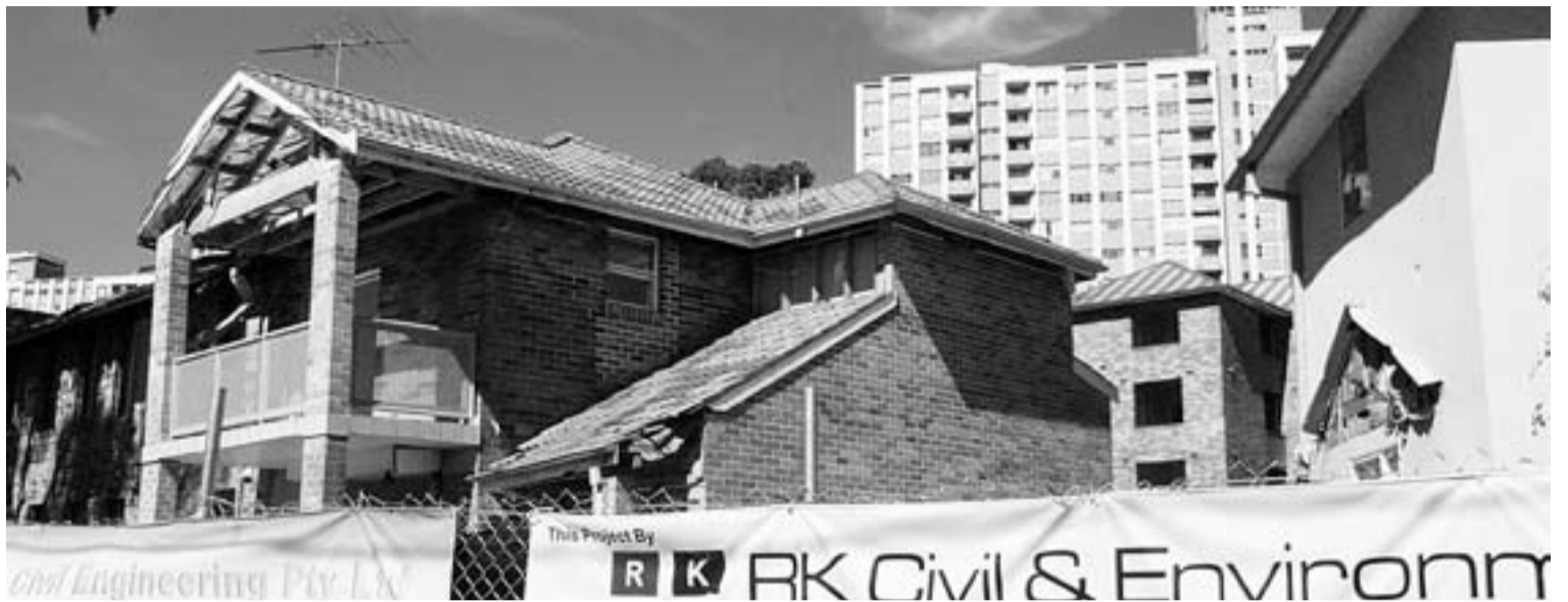
The demolition of units in Walker Street Photo: Ben Falkenmire
